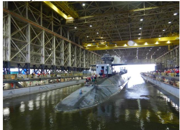
The Ohio-class ballistic missile submarine Tennessee enters the dry dock at the Trident Refit Facility in Kings Bay, Ga., on Feb. 1, 2021. (Elaine Rilatt/U.S. Navy)
