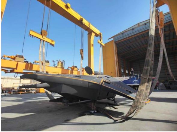
[Photo: Highland Systems]
