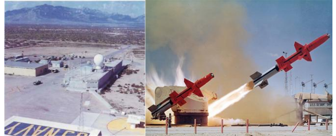
The facility from the air, with what looks like a box launcher installed for Sea Sparrow missile tests. Also, note the large trapezoidal building with GO NAVY on the top is the Talon assembly-magazine area just like the ones found on ships (Left image). Talos tests had to very lively affairs back in the 1950s (Right)!, USN
